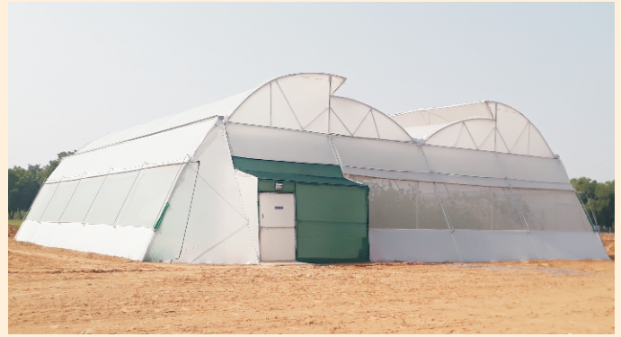
Naturally ventilated polyhouse
