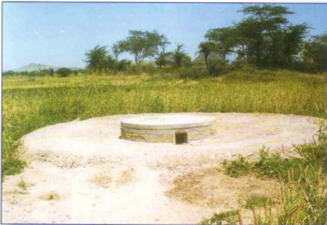
Improved tanka or 21000 liters capacity with catchment at Bambore (Distt. Jodhpur)
