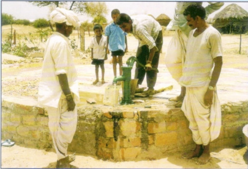
An improved multipurpose tanka (50,000 liters) with handpump for safe water withdrawal at a farmer's field - Kalyanpur (Distt. Barmer)
