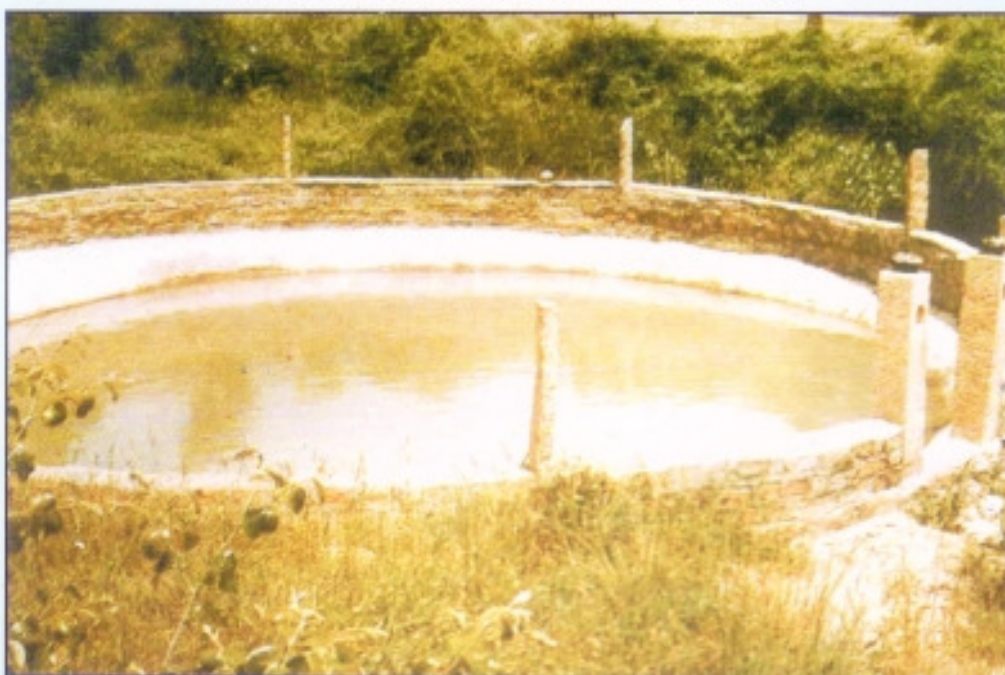
A open tanka of 271 m 3 capacity at farmer's field Jhanwar watershed (Distt. Jodhpur)
