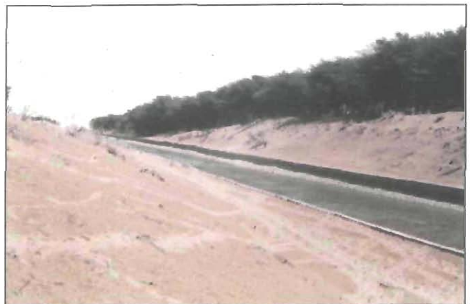
Plate 3. Encroachment of canal by deposition of wind blown sand at SBS 85 RD
